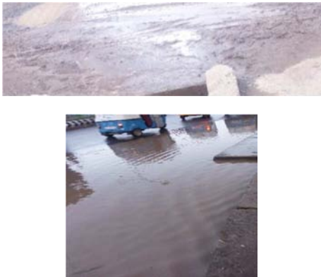
Figure 13. Improper connection of carriage way and side drainage structure.
