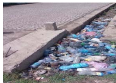
Figure 11. Deposited wastes in the drainage structure.
