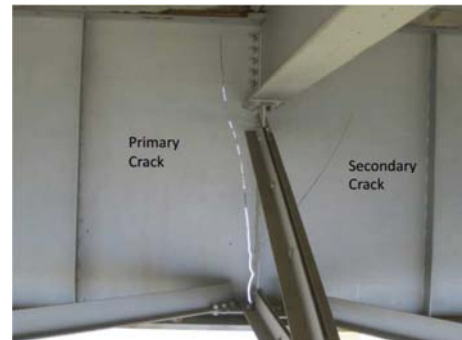
Figure 8. 2011 Diefenbaker Bridge cracks [17].
